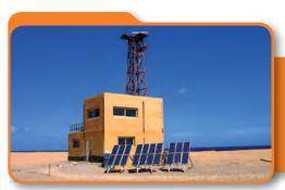
Photovoltaic systems are sometimes used in remote places where it is too expensive to use electricity cables.
